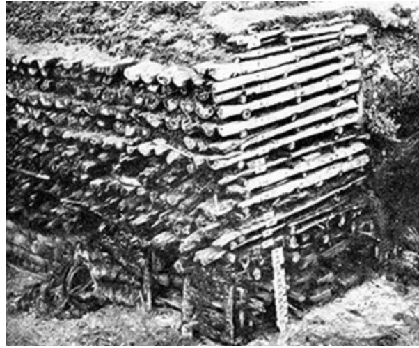
Fig. 3.29. Photograph of an excavation where one can see all 28 layers of the old paved streets of “Novgorod” on River Volkhov. Taken from [993], page 21.
